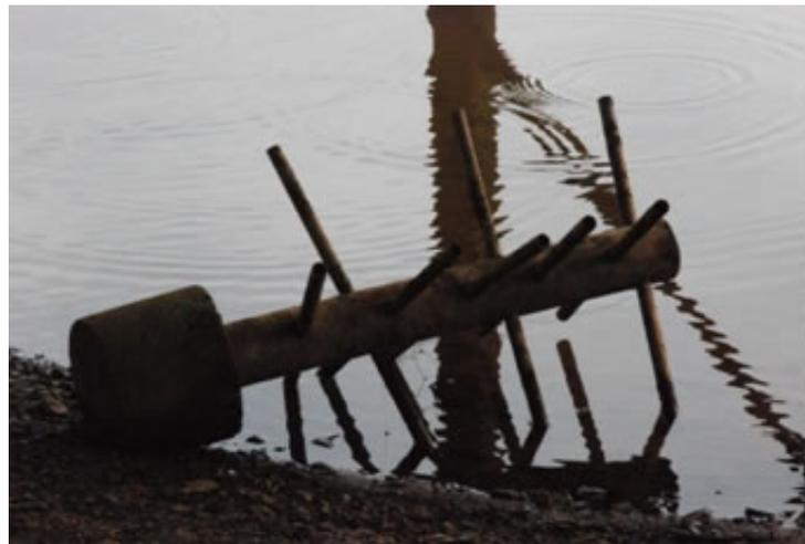
Here's a similar devise found under a pier in a cove off Dutch Second Creek; a 3" pipe imbedded in a concrete base, with 1" pipe stubs welded to the 3" core pipe.
